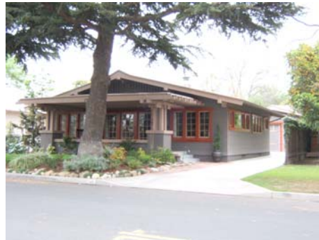
The Wilson House for Restoration
